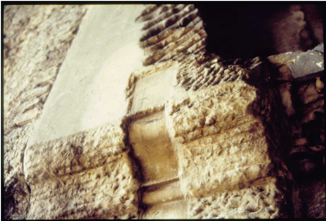
Figure 18: PR202_03_16: A sawn surface on the entablature of the Temple of Vespasian, Rome
