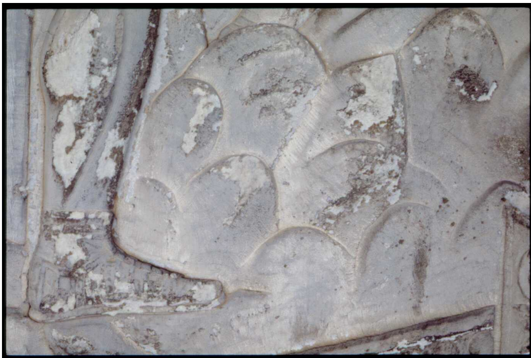
Figure 10: PR205_1_03_01: Detail of the background on the frieze of the Column of Trajan on which marks of the flat chisel are visible
