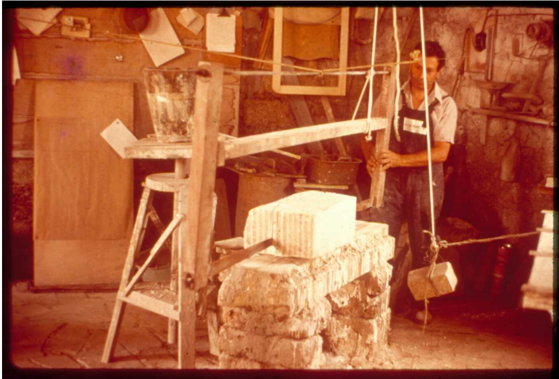
Figure 17: TE_5_2_1_1: Modern marble saw constructed in a traditional manner, Rome
