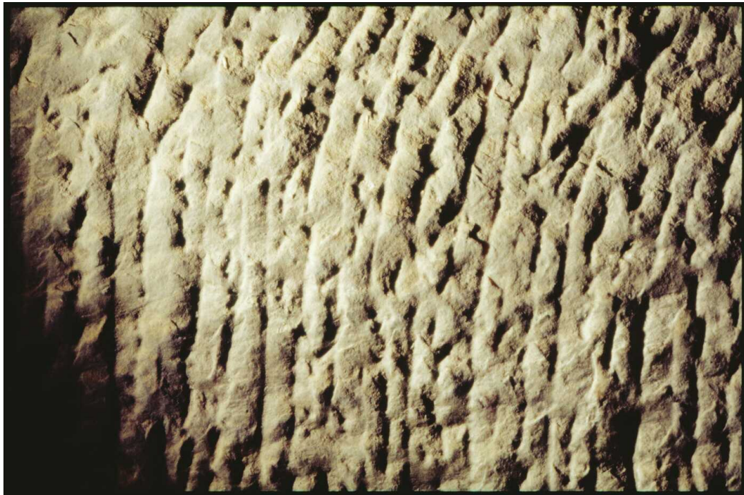
Figure 6: PR205_1_16_16: Point chisel marks on the interior of the Column of Trajan
