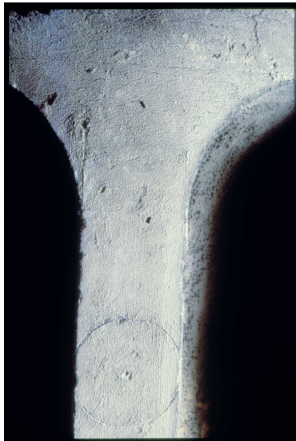
Figure 8: PR202_01_13: Guidelines on a column of the Temple of Vespasian, Rome
