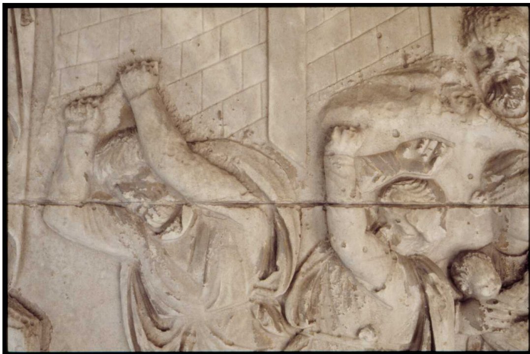
Figure 26: PR205_1_04_05: Detail of the Column of Trajan showing carving across a joint between drums
